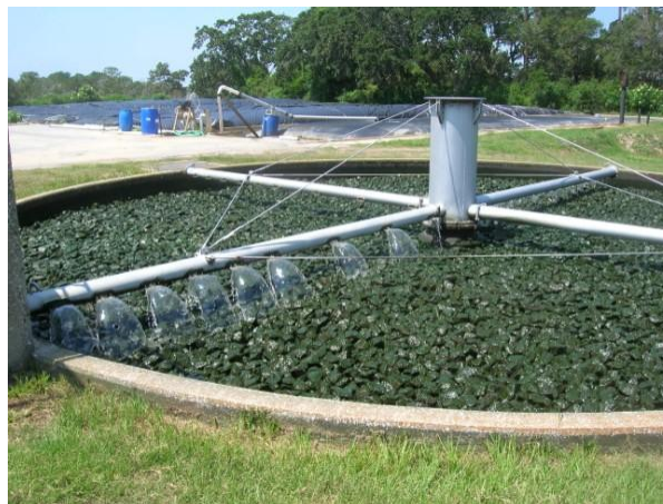
Fig: 4 Waste water Treatment by Trickling Filter.
