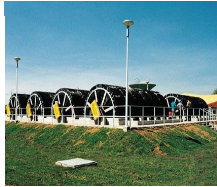
Fig: 5 Waste water Treatment by Rotating Biological Contractor
