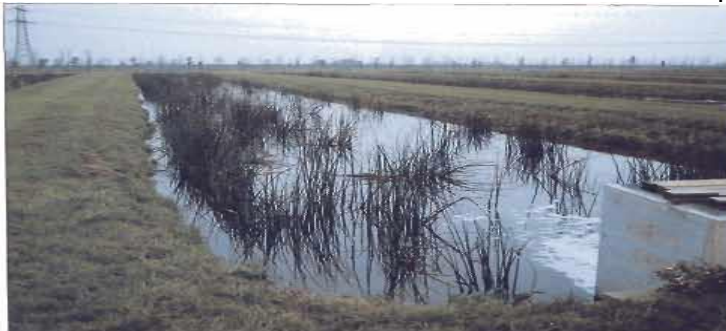
Fig: 6 Treatment of Waste water in ditches planted with ( Scirpus lacustris ) (Source: Hans Brix and Hans-Henrik Schierup, 1989)
