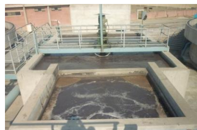
(b) Digester Tank (Sludge)
