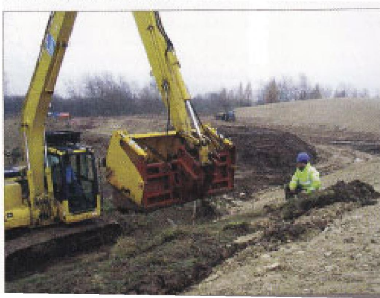
Figure 7. Placing turfs on the new landscape bund at Boston Spa
