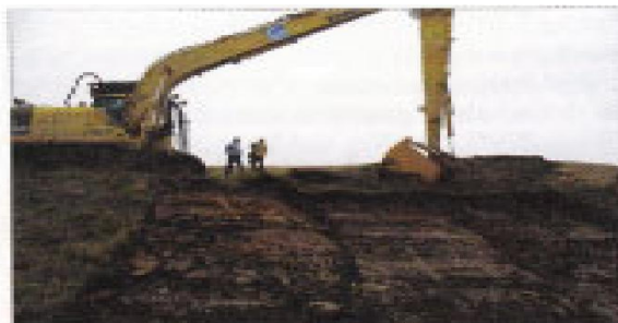
Figure 6. Removing 1 x 0.5 x 0.3 m turfs from the Boston Spa site with a modified bale-cutting bucket in spring 2006
