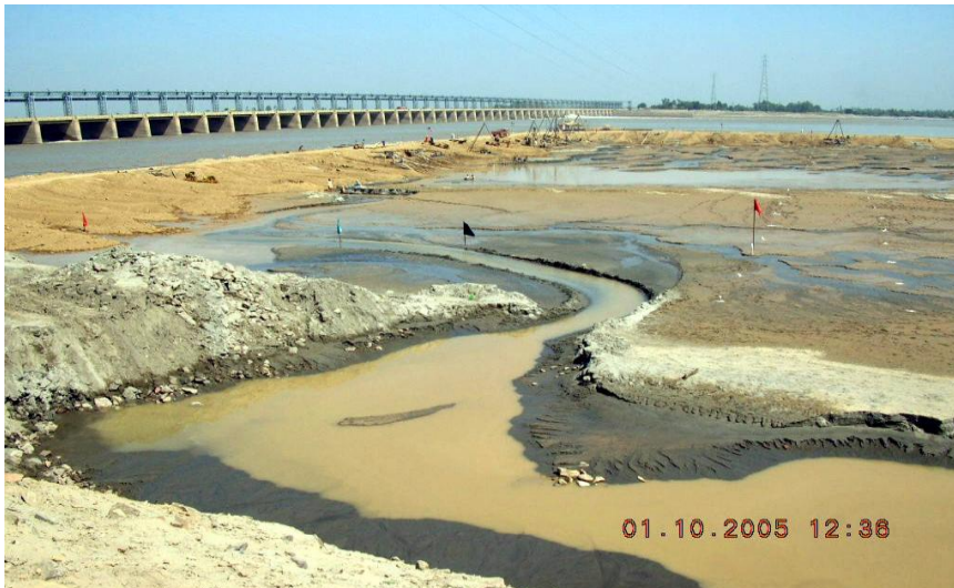
Cofferdams – unwatering of enclosure
