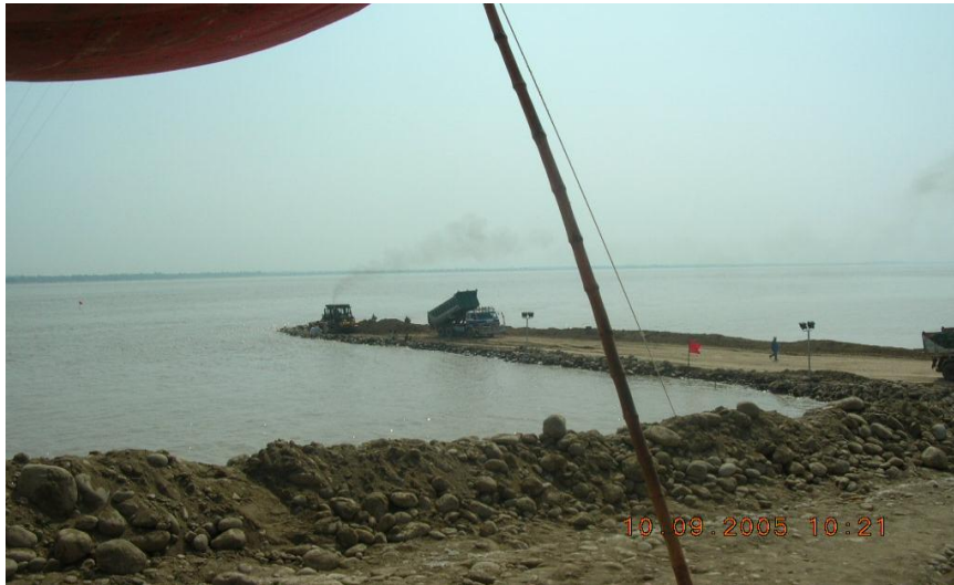
Start of coffer dam
