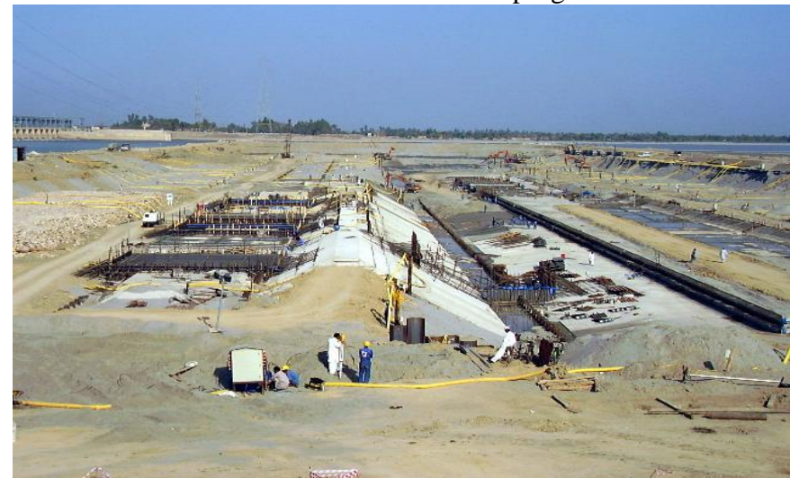
Sub-weir Construction in progress
