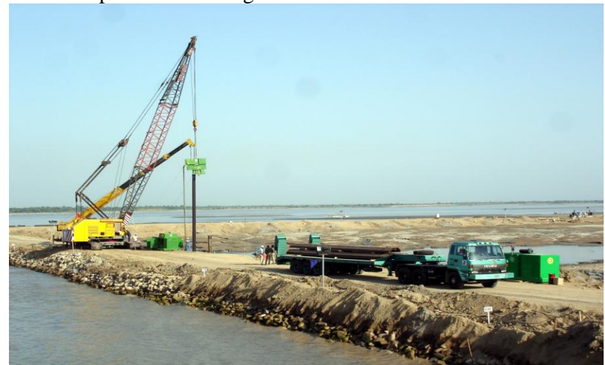
Cofferdams - Sheet Piling in progress
