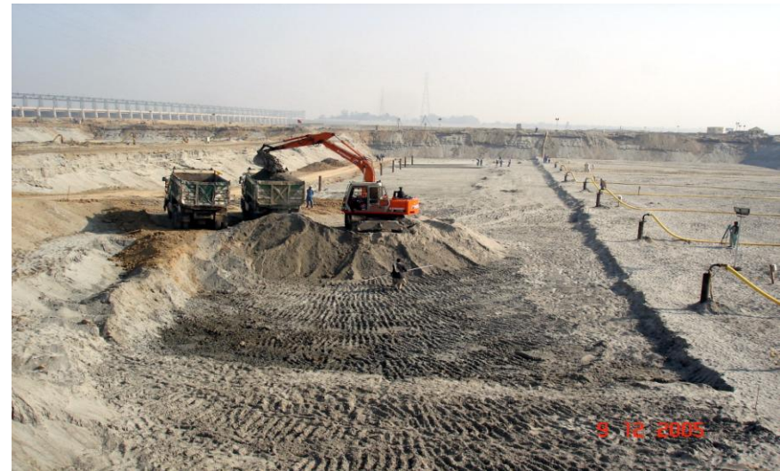
Cofferdams - Subweir dewatering wells installed with simultaneous excavation in progress
