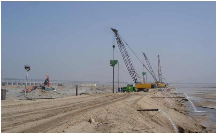
Sheet Piling in the cofferdams with simultaneous dewatering
