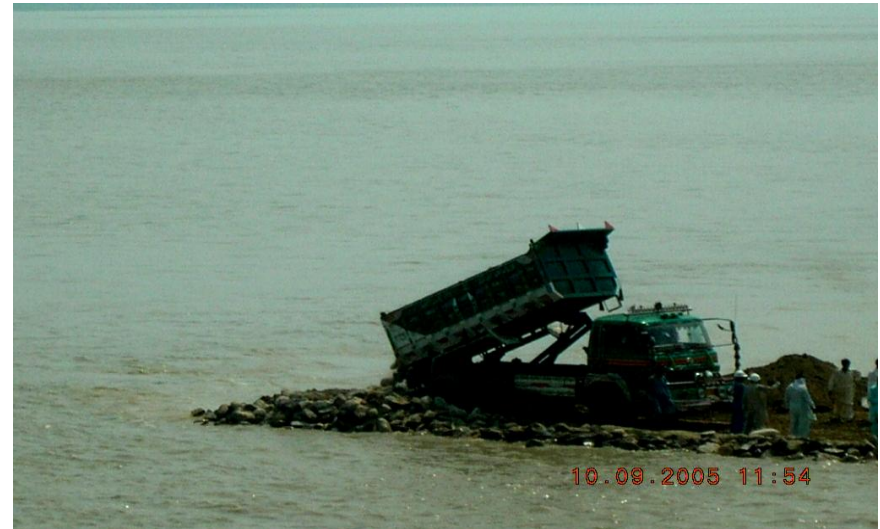
Dump truck unloading stone at the nose of the cofferdam
