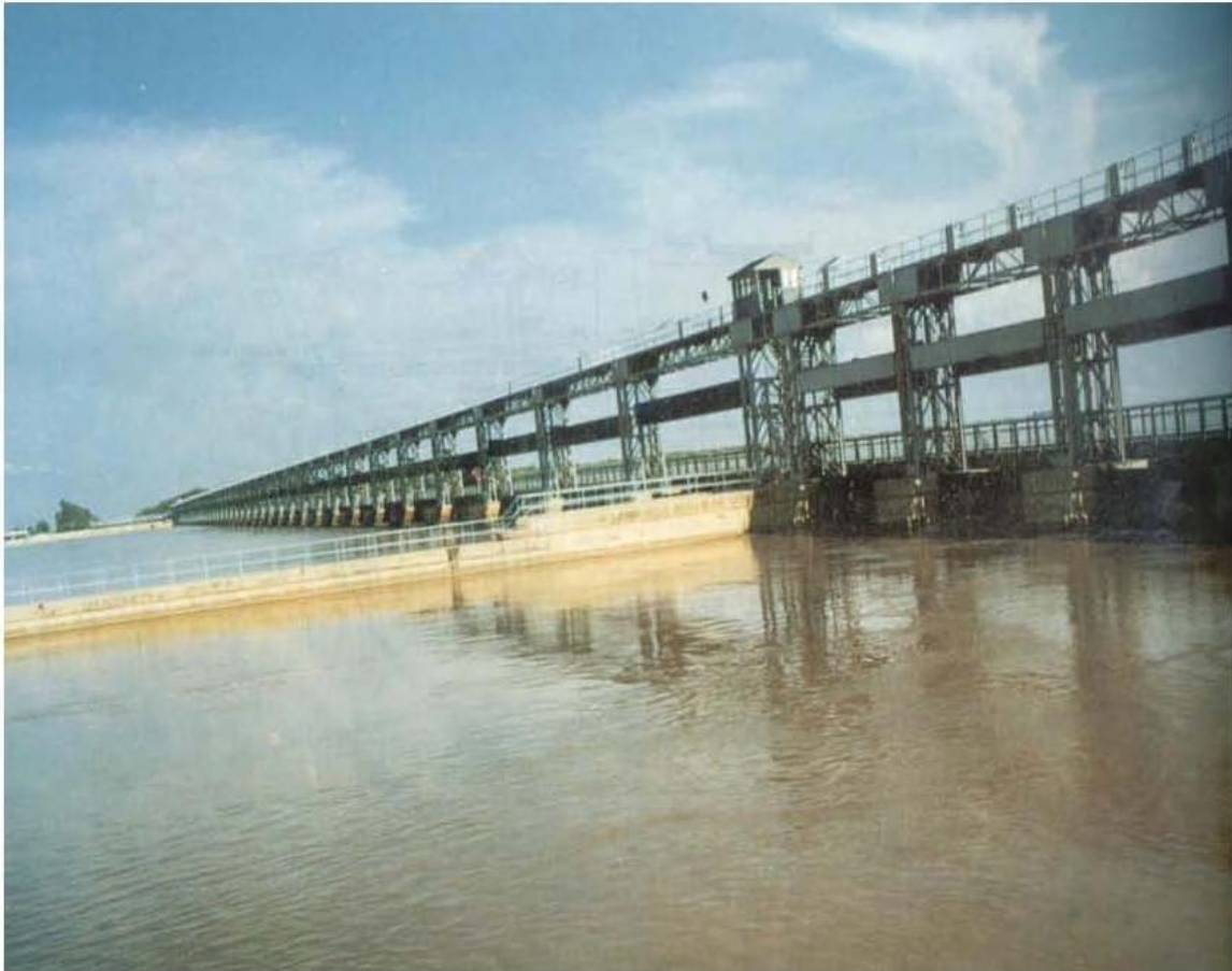
Figure 1: Upstream View of the Barrage
