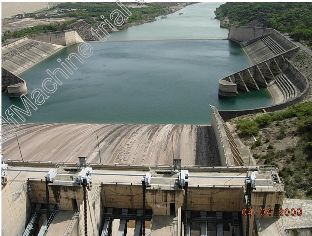
Down Stream View of Main Spillway Showing Chute & Stilling Basin
