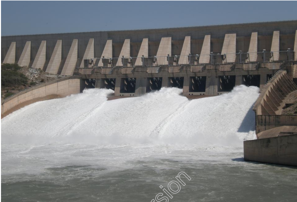
General View of Main Spillway after Completion
