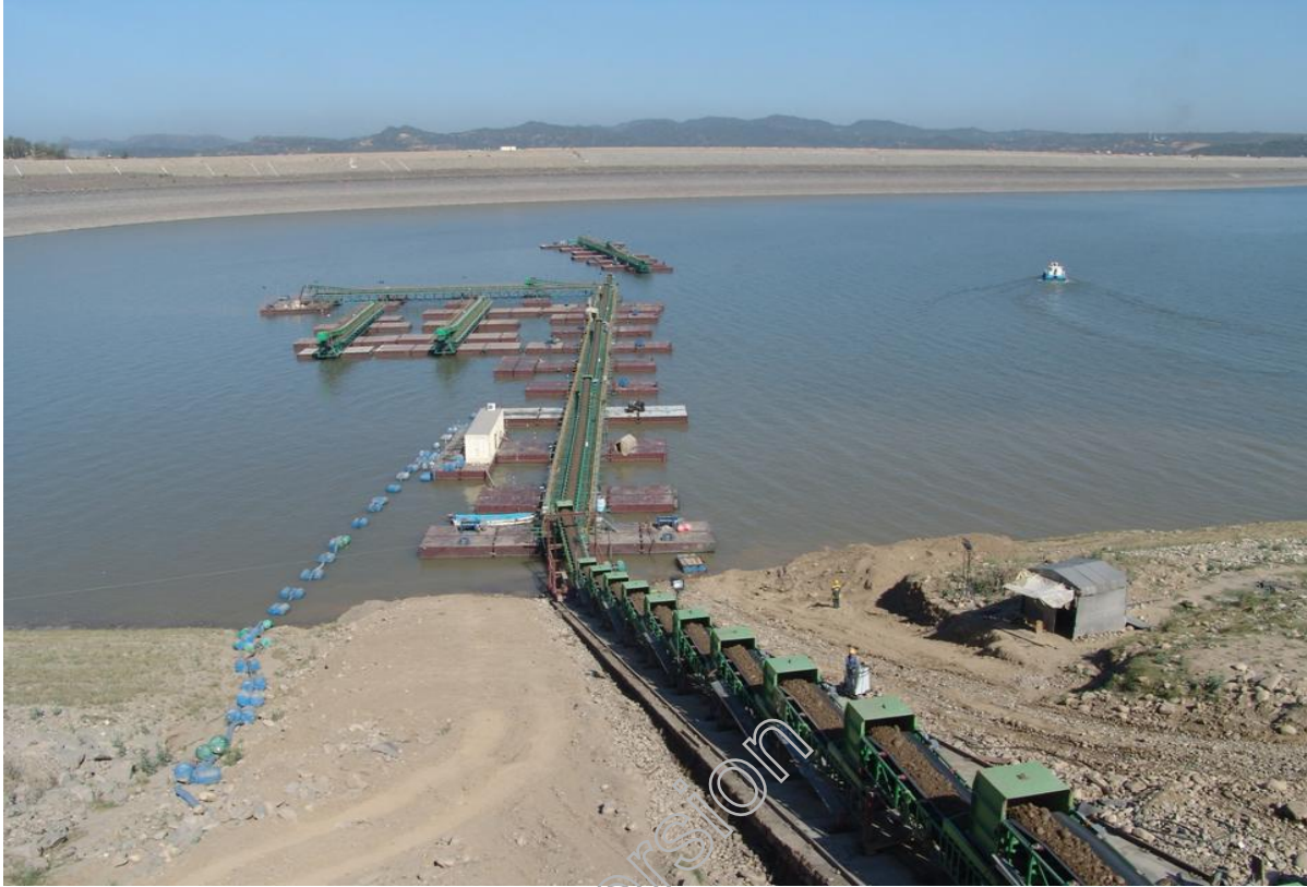
Under Water Filling at Upstream Intake Toe Weight is in Progress
