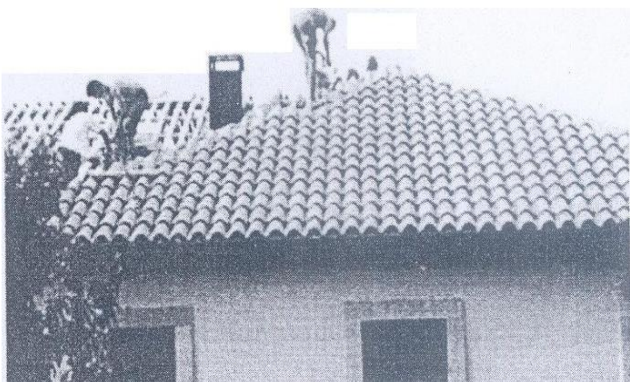
Fig-5: Construction of tile roof in Czech Republic
