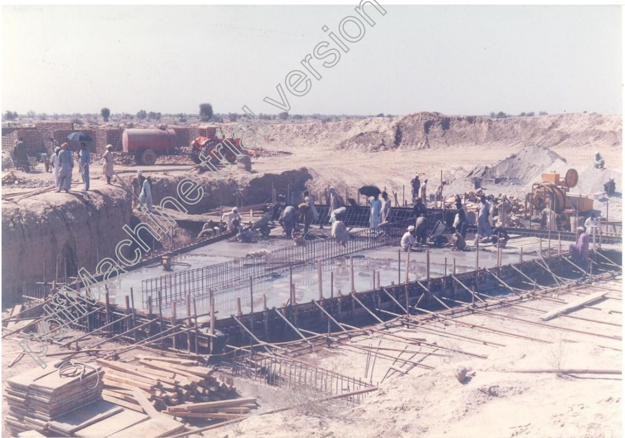
Fig-6: Placing of Concrete by labour force on a Site in Pakistan
