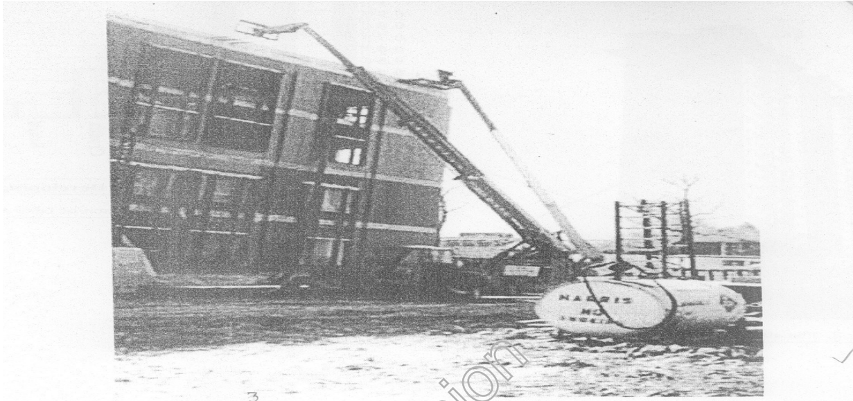
Fig 3: Use of lifting equipment on U.S. Construction Site
