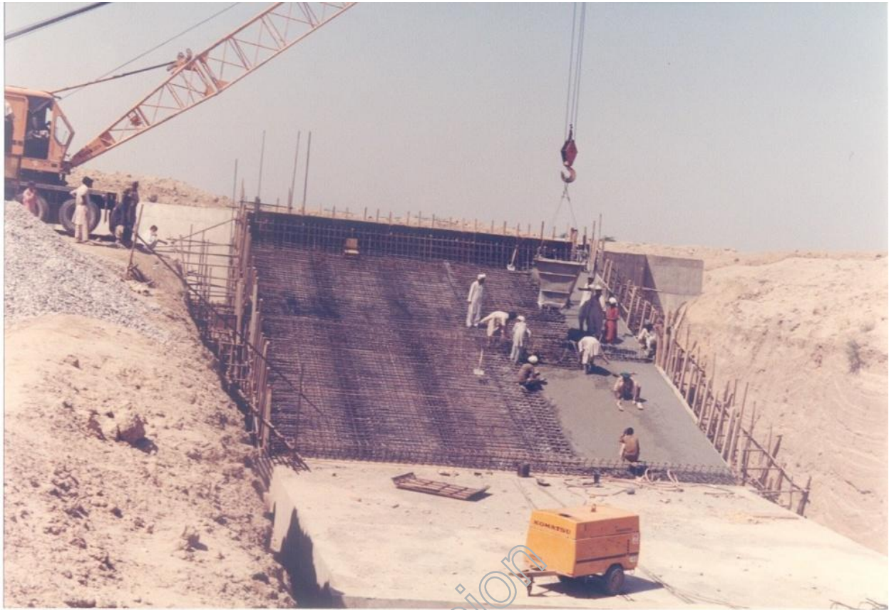
Figure 1: Placing of Concrete by Crane at Chashma Right Bank Canal, Pakistan
