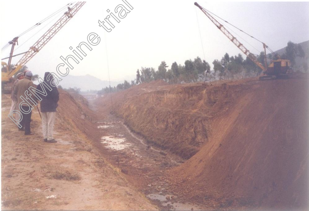
Fig 2: Carrying out under-water Excavation by Draglines on Swabi SCARP, Pakistan
