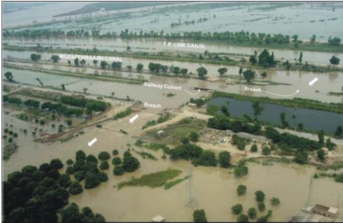
Figure 14: Breach of T.P. Link and Muzaffargarh Canals
