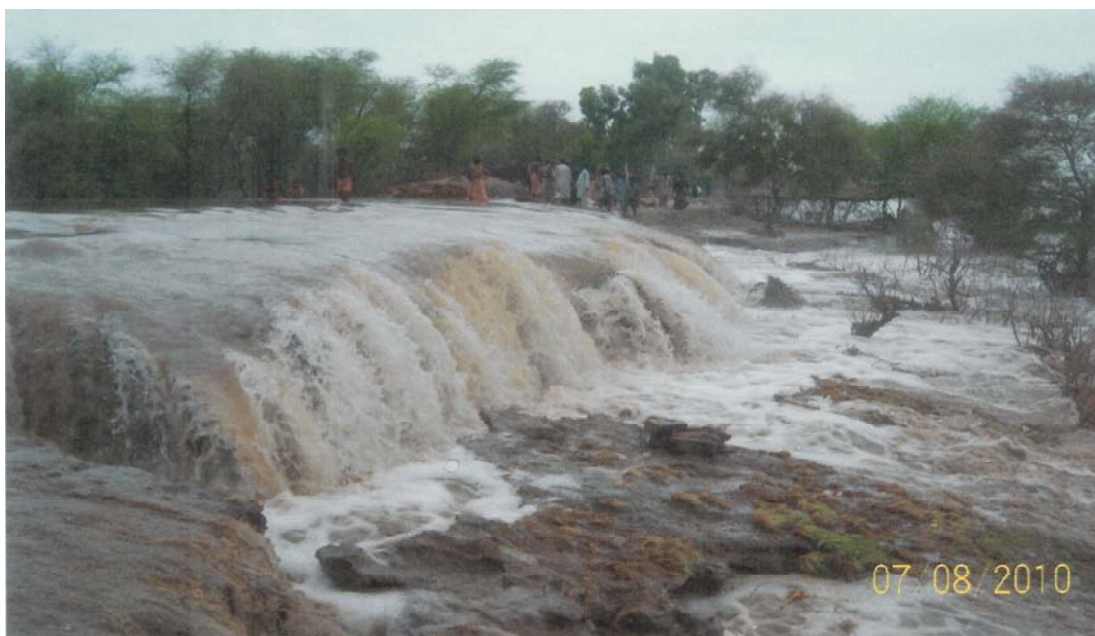
Figure 16: Initial Stage of Breach of Tori Flood Bund in Sindh Province
