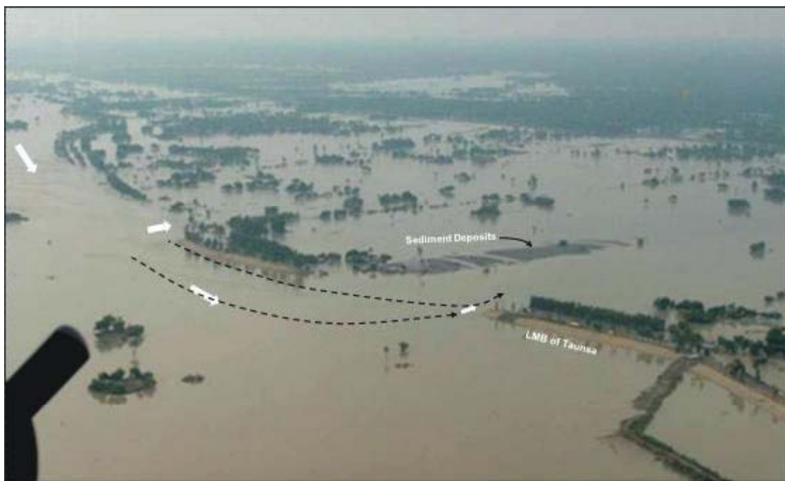
Figure 13: Breach of LMB of Taunsa Barrage
