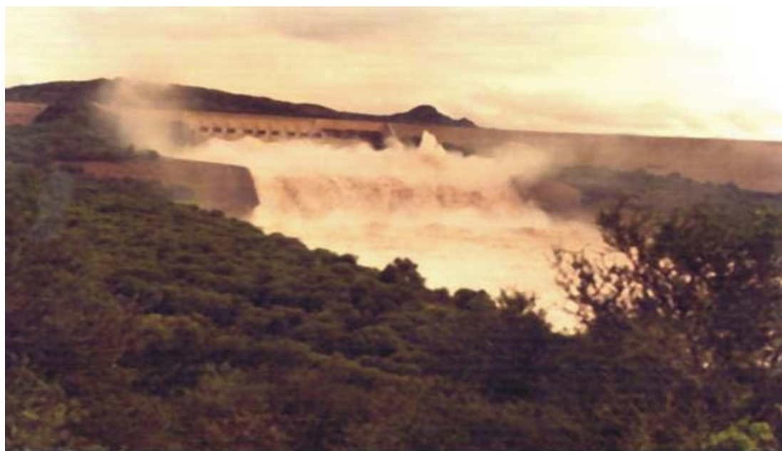
Figure 12: Operation of Mangla Dam Spillway at discharge of 1 million cf
