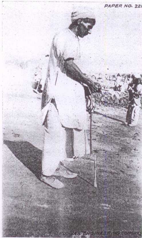
Photo No. 5. Testing Joints.
