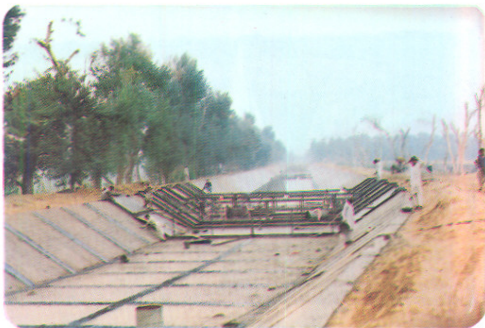
Alternate Panels of P.C.C. Lining being laid in 6-R (Hakra) Disty:
