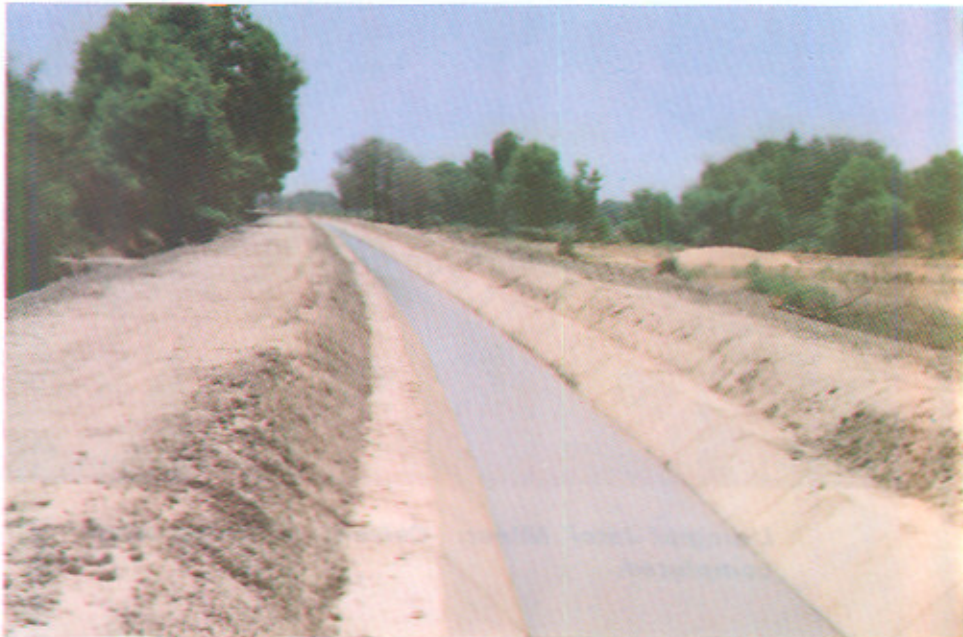
Finished P.C.C. Lining View of Old Ketu Minor at RD. 5+000
