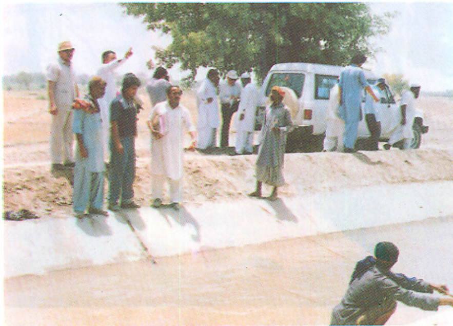
Running of Salehpur Minor after completion of Lining.
