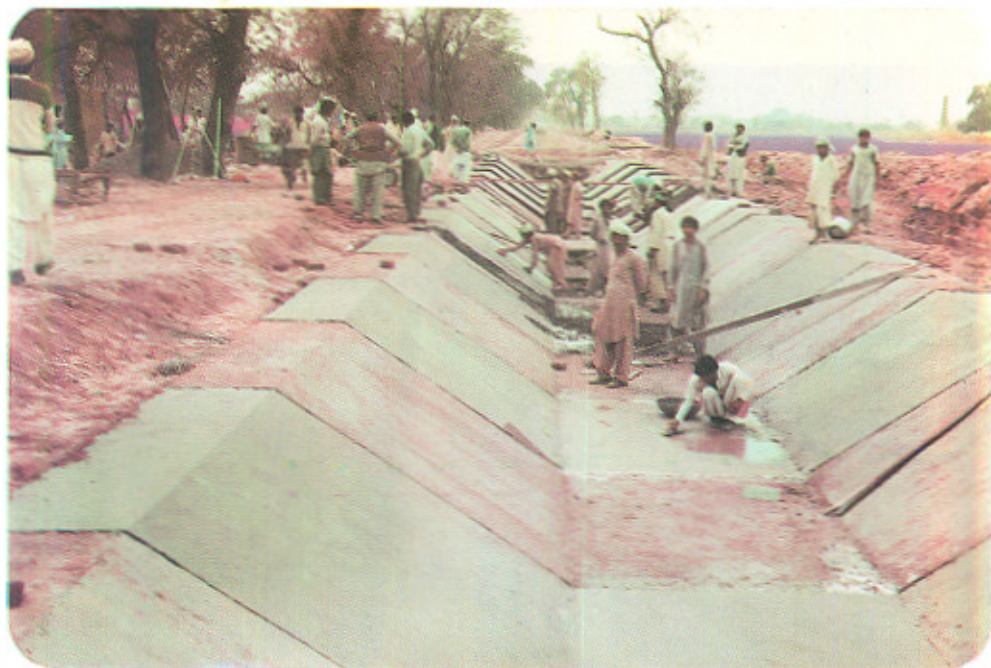
. LINING WORK ON NIAZ-BEG DISTRIBUTARY IN PROGRESS
