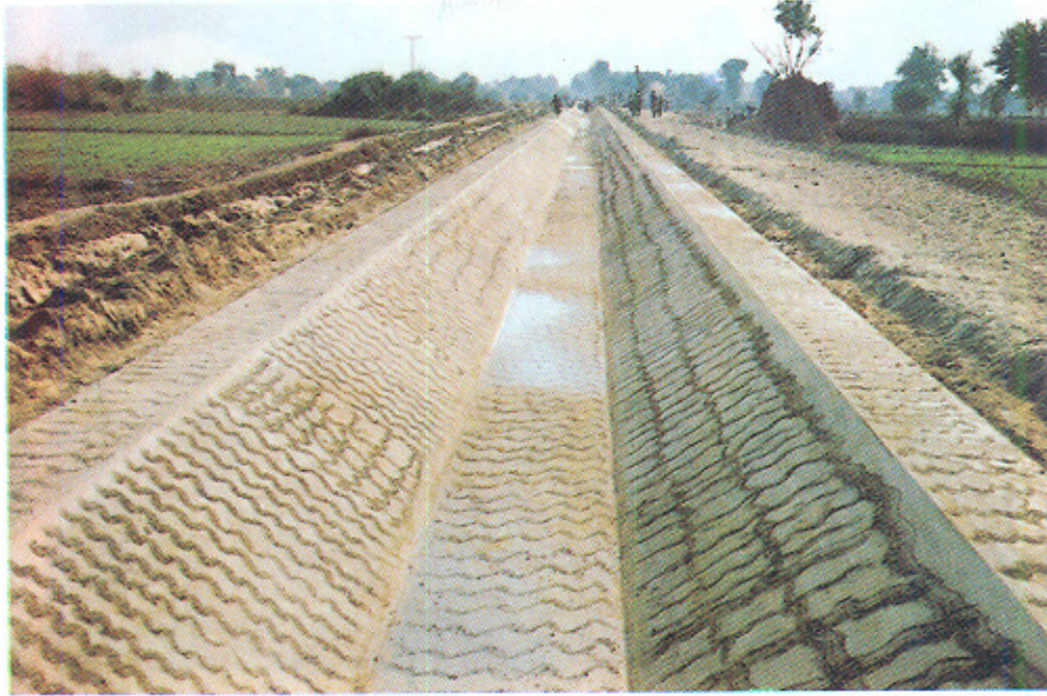
Lining of Dewan Minor. Cement Plaster completed-RD 5+000.
