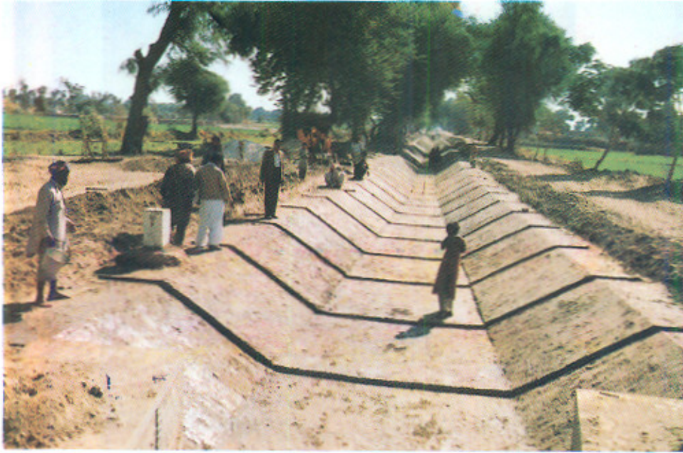
Lining of Jatoi Minor. Formation of Bed/Slopes & Excavation for Profiles completed.
