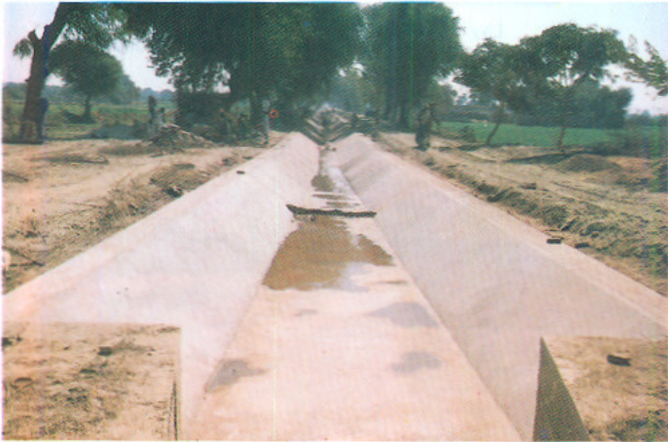
Lining of Jatoi Minor. Cement Concrete work completed.
