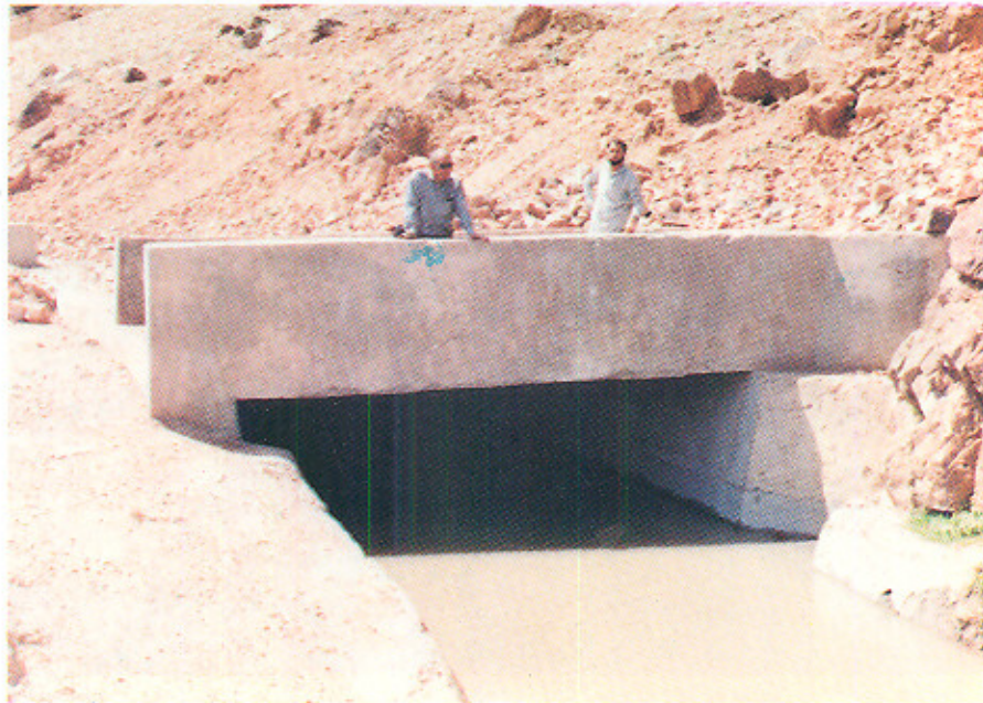
A view of Canal covering in the reach R.D. 0+700 to 1+000.
