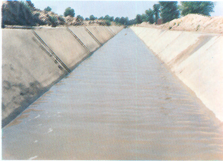
P.C.C. Lining on Niaz Beg disty. Downstream R.D. 134.
