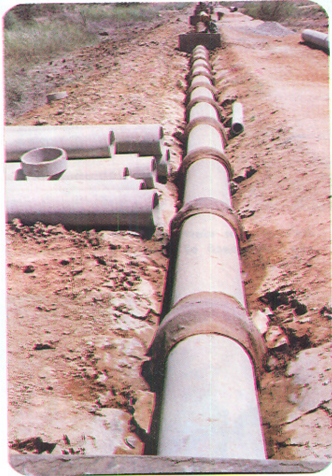
PIPE LINING OF MINOR NO. 1 DOWN STREAM BRIDGE RD. 2980
