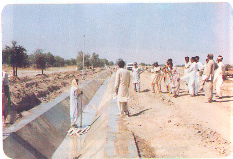
A FINISHED LINED REACH BEING CHECKED FOR LEVEL AND GRADE
