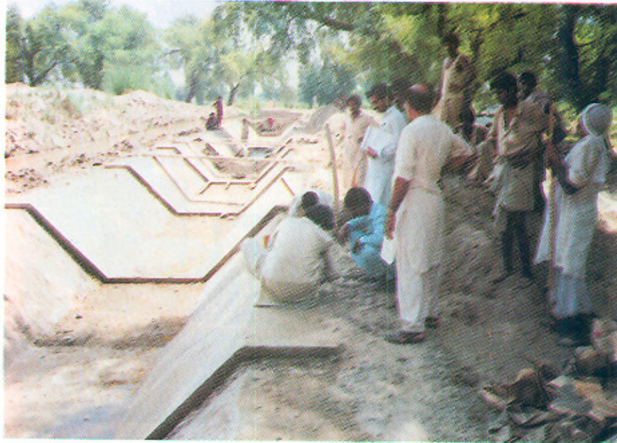
P.C.C. Lining Work in progress on a Channel in Pakpattan Sub-project.
