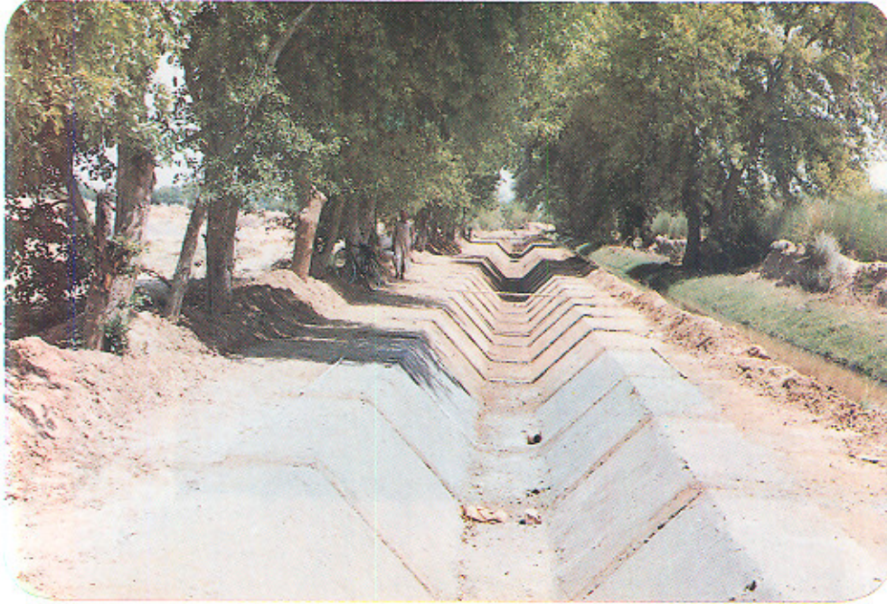
A CHANNEL PRISM WITH LAYER OF LEAN MORTAR VISIBLE IN THE FOREGROUND BAYS WITH EARTHEN SECTION BEYOND, ORIGINAL SECTION RUNNING FOR FEEDING CROPS.
