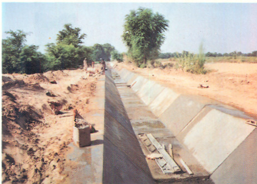
Finished P.C.C. Lining on IR|IL|6-R sub-minor.
