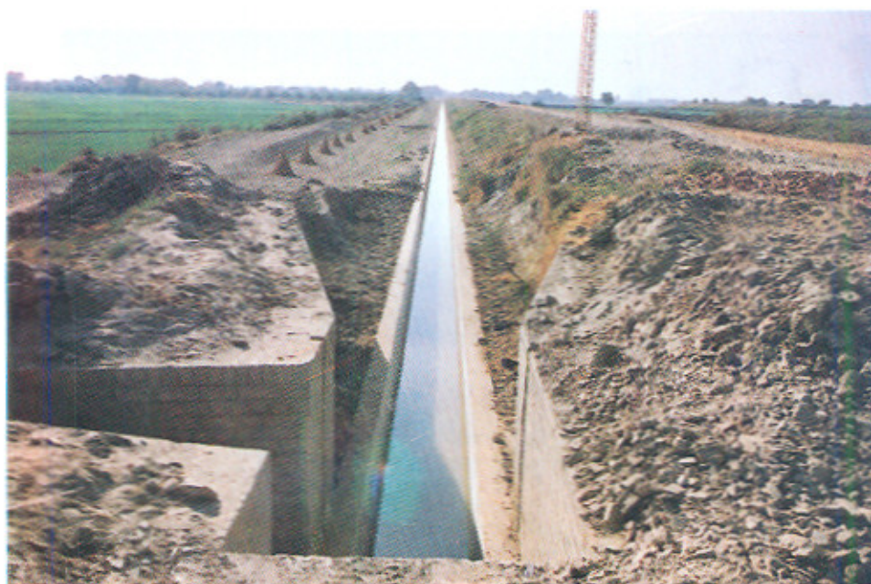
Lining of Mahessar Minor after Completion-RD 6+000.
