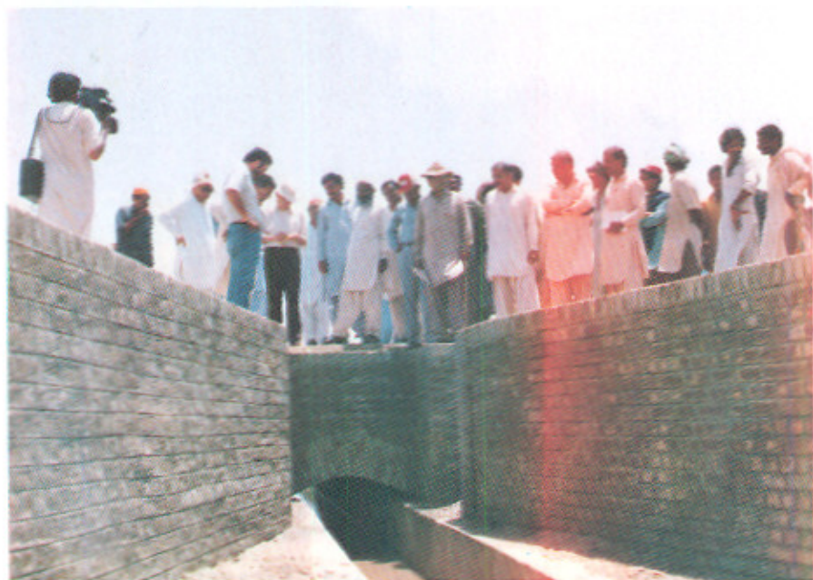
Bund Sluice in Head Reach on Mahessar Minor.
