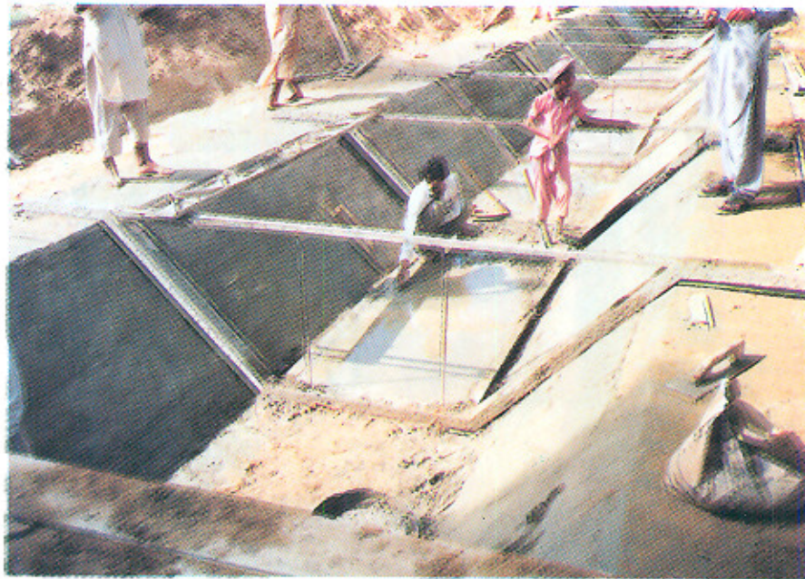
P.C.C. Lining in progress on Niaz Beg distribu. tary.
