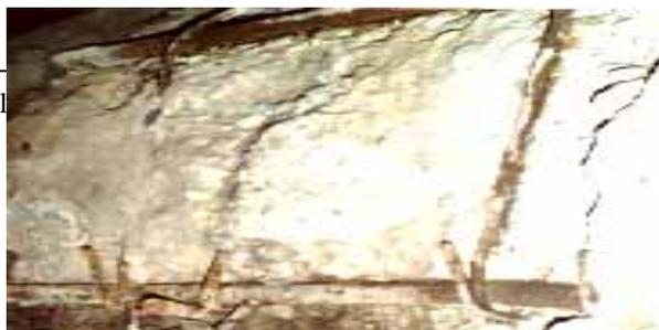
Fig. 1. Fall of concrete cover due to corrosion of the steel reinforcement
