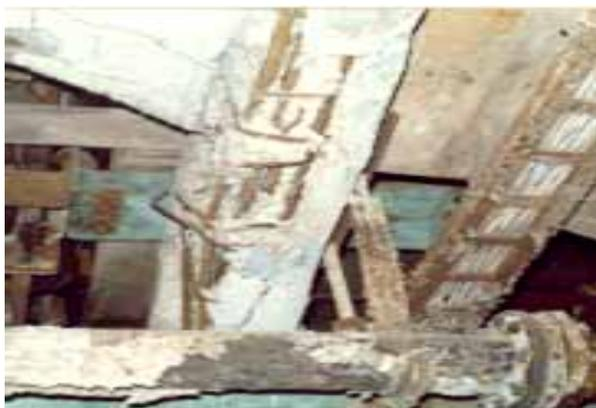
Fig. 2. Corrosion of the Steel in Concrete
