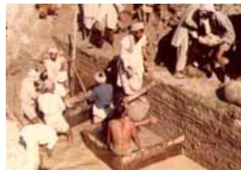
Concreting through caissons along the cracks
