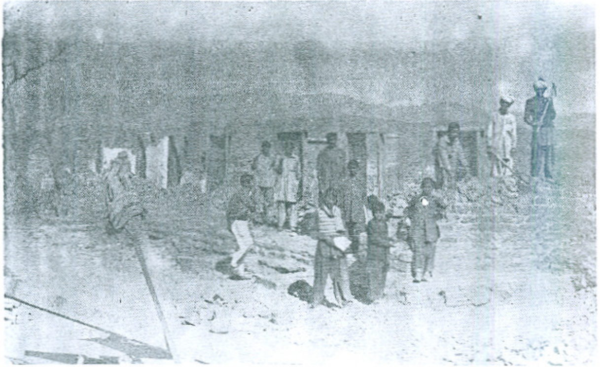
Plate No. 7 Extensively damaged part of Kuri School being demolished.
