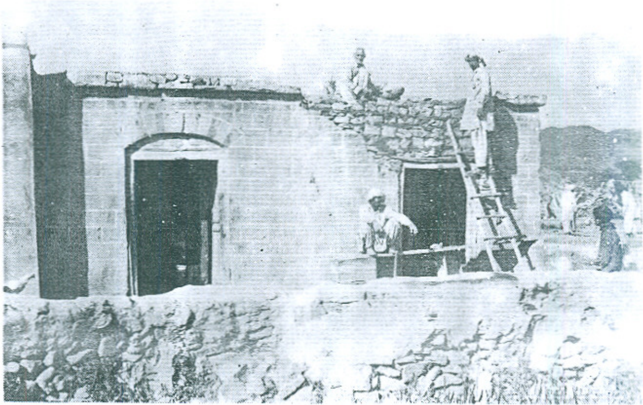
Plate No.1 Partial collapse & cracks in houses being repaired-Athal
