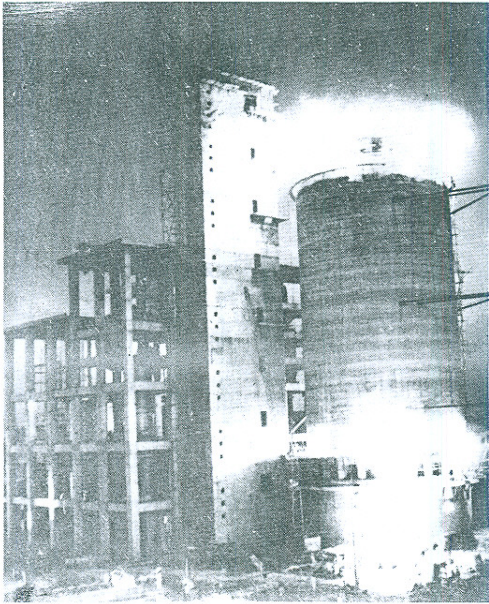
Fig. 21. Illumination for Night Work at NP Prilling Tower
