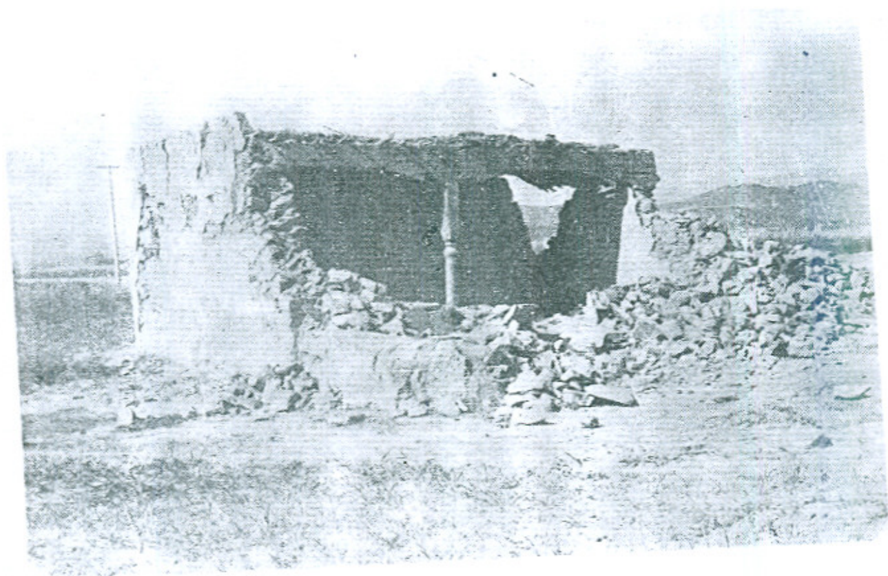
Plate No. 2 Collapse of a House near Pind Begwal
