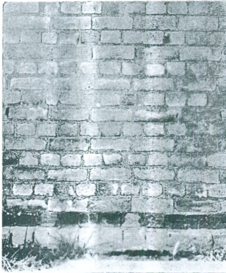
PLATE 4 No Deterioration when Bitumen Impregnated Bricks were used for Impervious Course.
