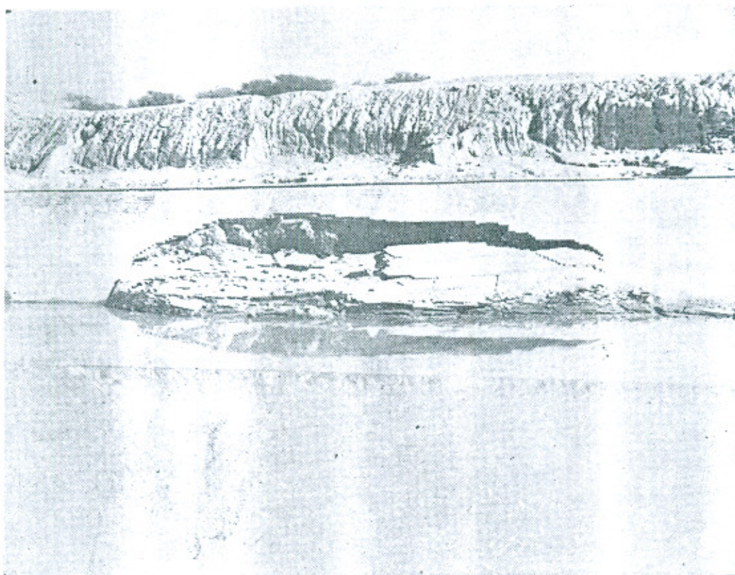
Damage to canal lining by pressure of wet soil.
