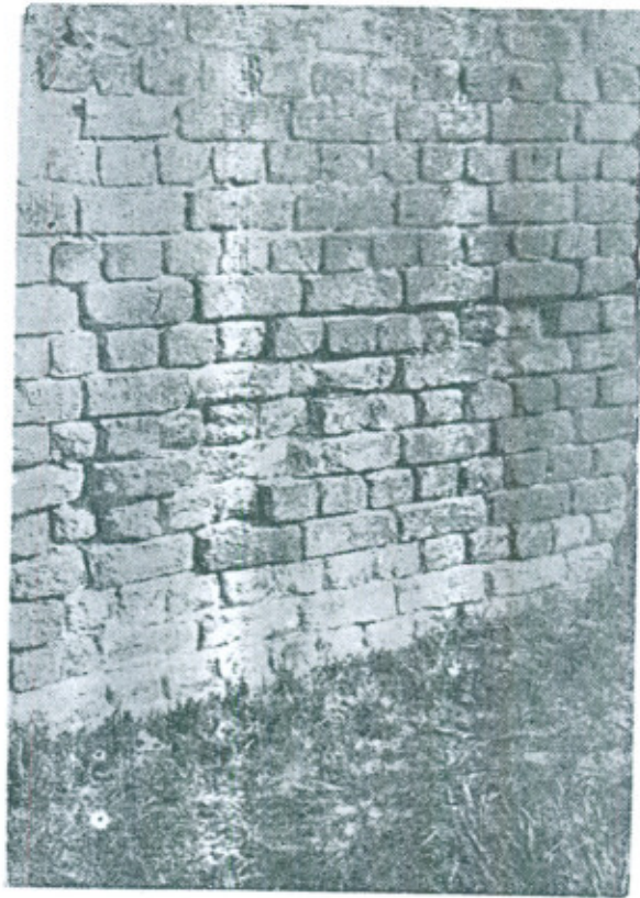
PLATE 4 No Deterioration when Bitumen Impregnated Bricks were used for Impervious Course.
