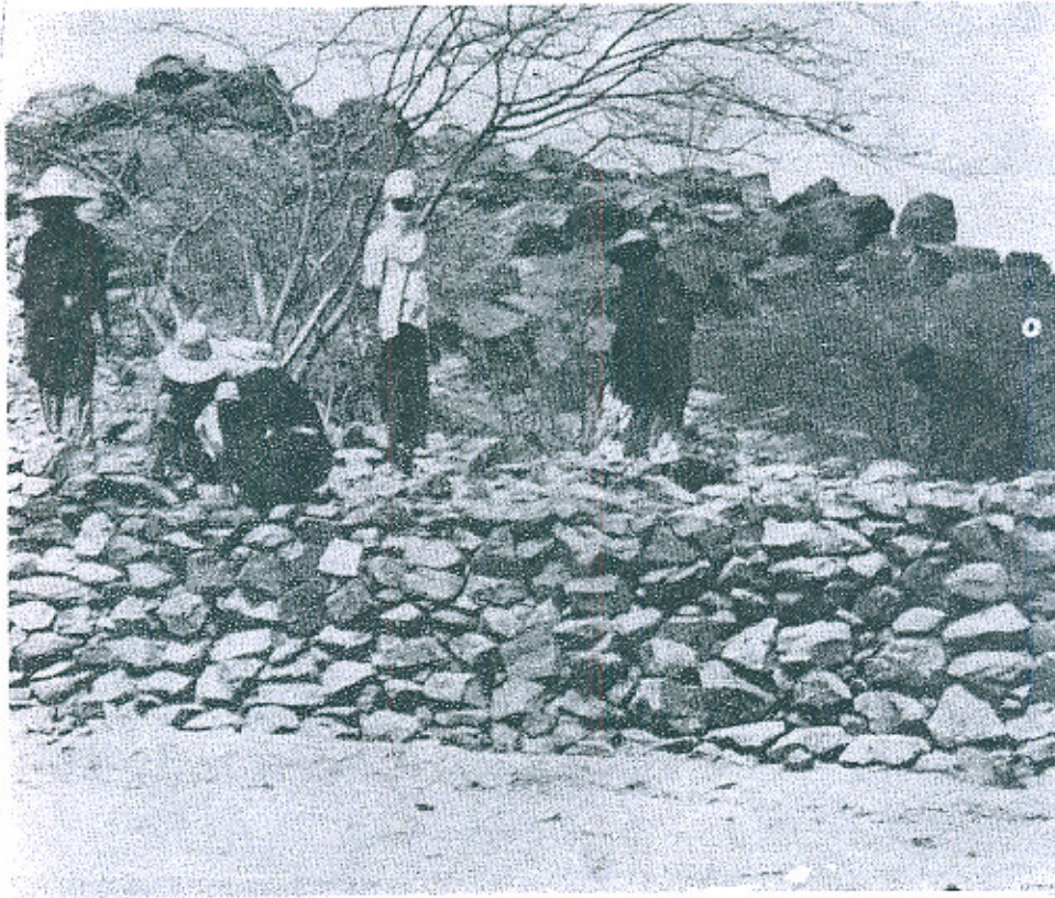
FIGURE 19 In 1972 near the small town of Tchirozerine (close to Agades), Niger, West Africa, Touareg nomads build a rock wall to capture flood waters. The soils here absorb little moisture, and the rainfall runs away in flash floods. Using stones gathered from the fields, Touareg workers built eight 1-m-high walls across the plains so that rain is retained, and absorbed by the soil. When summer showers fell in 1973, the water retained by stone dams and walls flooded nearly 1 square mile on the plain and grass flourished—extraordinary events in that area. (Oxfam-America)
