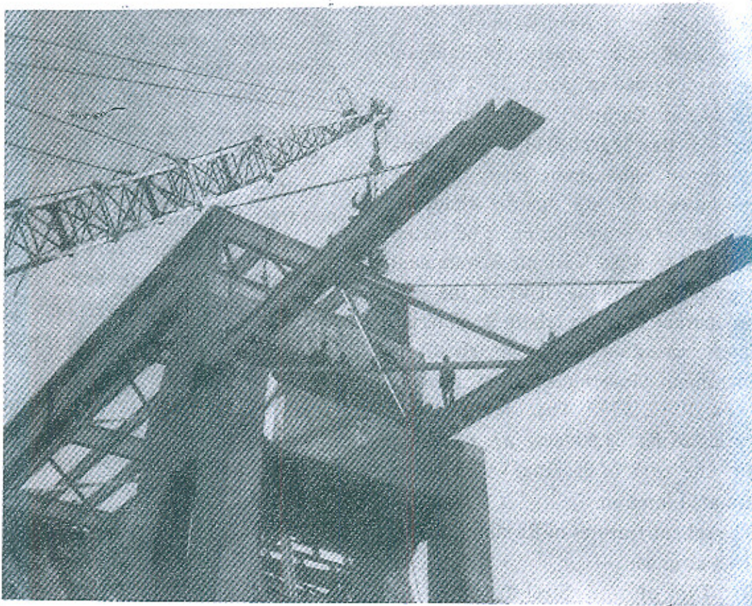
Launching of Bridge between left abutment and pier 3.
