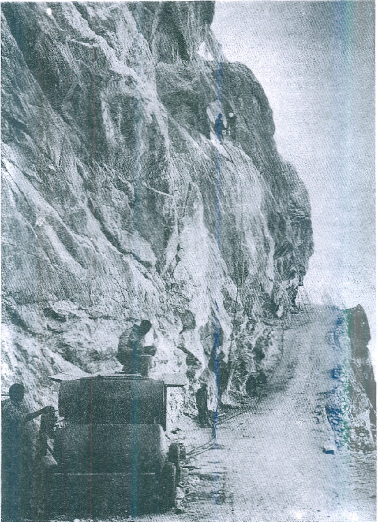
Drilling work in progress on Karakoram Highway
