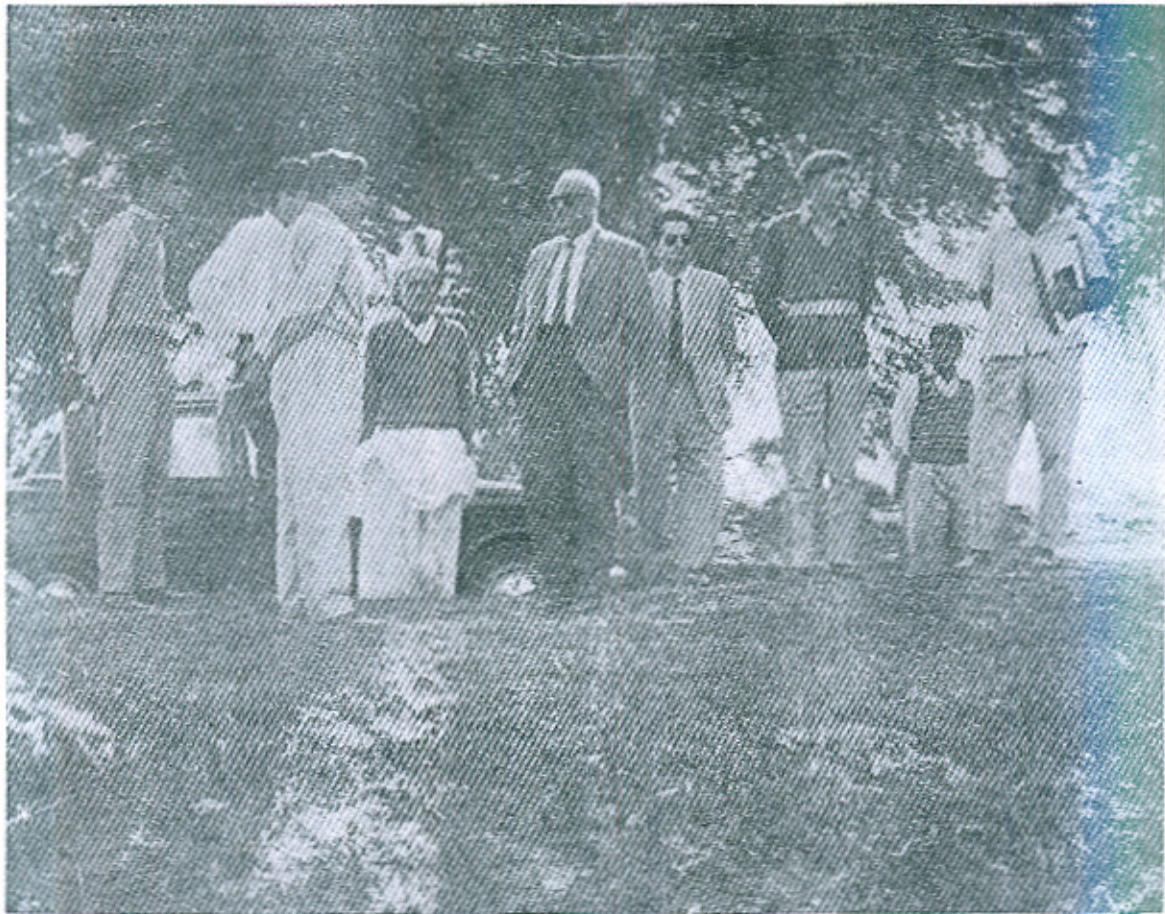
Mian Alim-ud-Din, Ex-Chief Engineer, Irrigation Lahore Zone, giving instructions to Incharge Officers and the contractor at site during Remodelling of Dipalpur Canal
