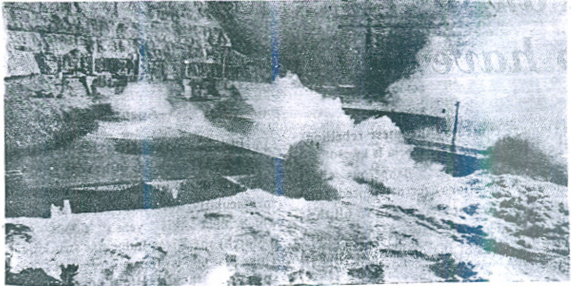
This perspective, based on site drawings produced from the divers' surveys, shows part of the damage to stilling basin 3. Four monoliths of the dividing wall (right) are held only by the keying action of the joints.
