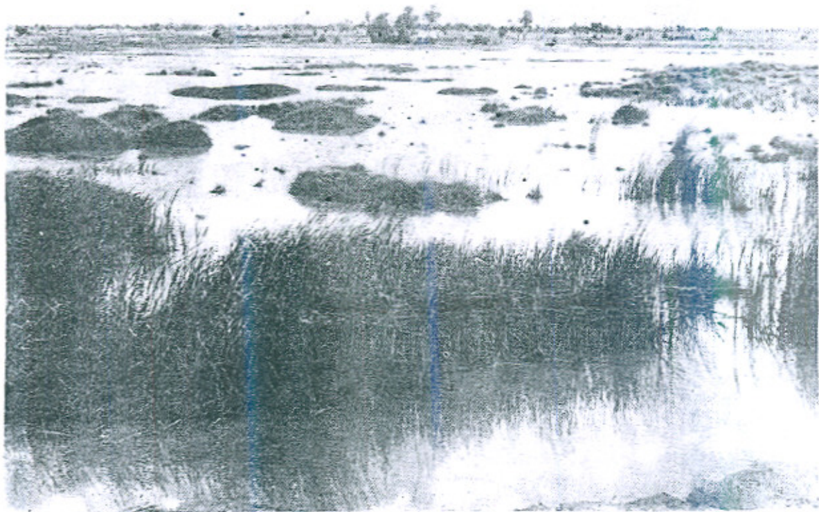
A view of waterlogged land along Left Bank of T.S. Link
