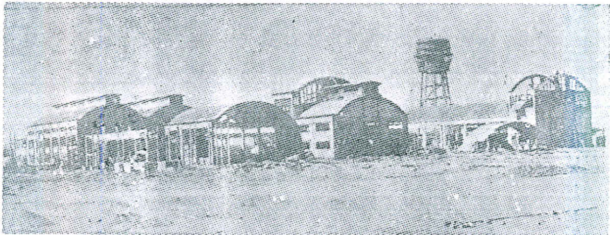
United Chemicals Factory Under Construction at Kala Shah Kaku. Design and Construction by Conforce
