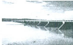
A view of Tausa Barrage Project
