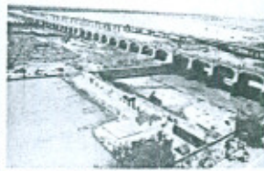
Sukkur Barrage Rehabilitation Project Completed Upstream Coffor Dam
