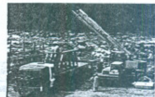
Allai Khwar Project: Off-Loading of Contractor's Construction Equipment at Power House
