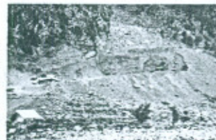
Duber Khwar Project: Excavation
