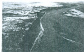
A view of Irrigation Channel under Merowe Irrigation and Dam Project in Sudan
