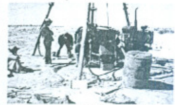
Drilling for Geo-technical Investigations in Progress with Rotary Rig in the Extension of Pat Feeder Canal Project Extension Area.
