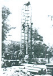
WASA Project -Tubewell boring in Progress
