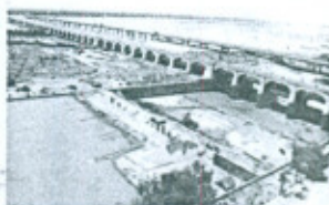
Sukkur Barrage Rehabilitation Project Completed Upstream Cofferdam
