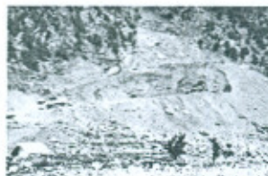
Duber Khwar Project: Excavation
