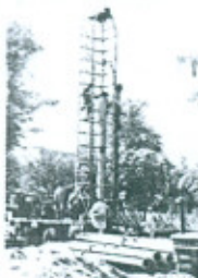
WASA Project - Tubewell boring in Progress
