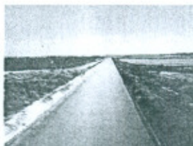
A view of Concrete lined Canal under the Revamping/Rehabilitation of Irrigation and Drainage Systems in Sindh Project
