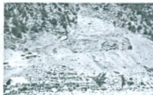
Duber Khwar-Project: Excavation
