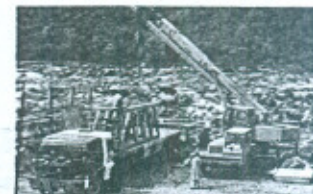
Ailal Khwar Project: Off-Loading of Contractor's Construction Equipment at Power House
