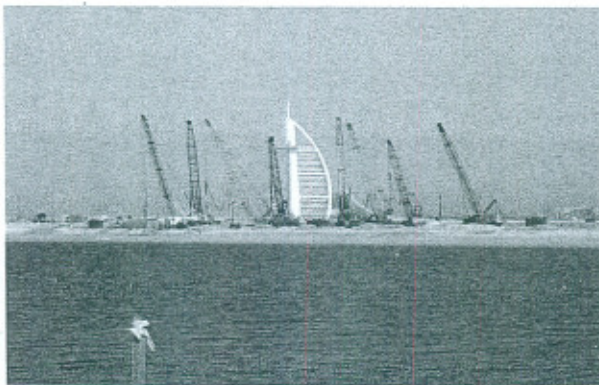
Fig: 9 Sand Compaction at Palm Jumeirah-Dubai
