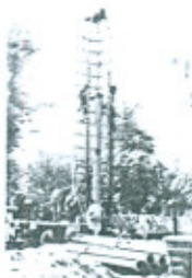
WASA Project - Tubewell boring in Progress
