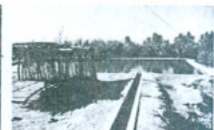
A view of Lined Watercourse in Balochistan
