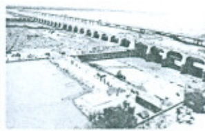
Sukkur Barrage Rehabilitation Project Completed Upstream Cofferdam
