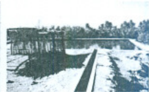
A view of Lined Watercourse in Balochistan
