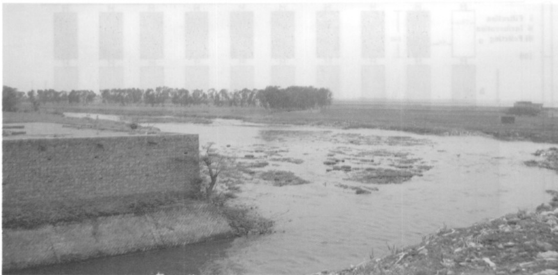
Fig. 3. The high risk piece of land between the sewage channel (outfall) and the active channel of river Ravi proposed for the treatment plant. This photograph was taken in March 2005; it is showing the rapid pace of encroachment.
